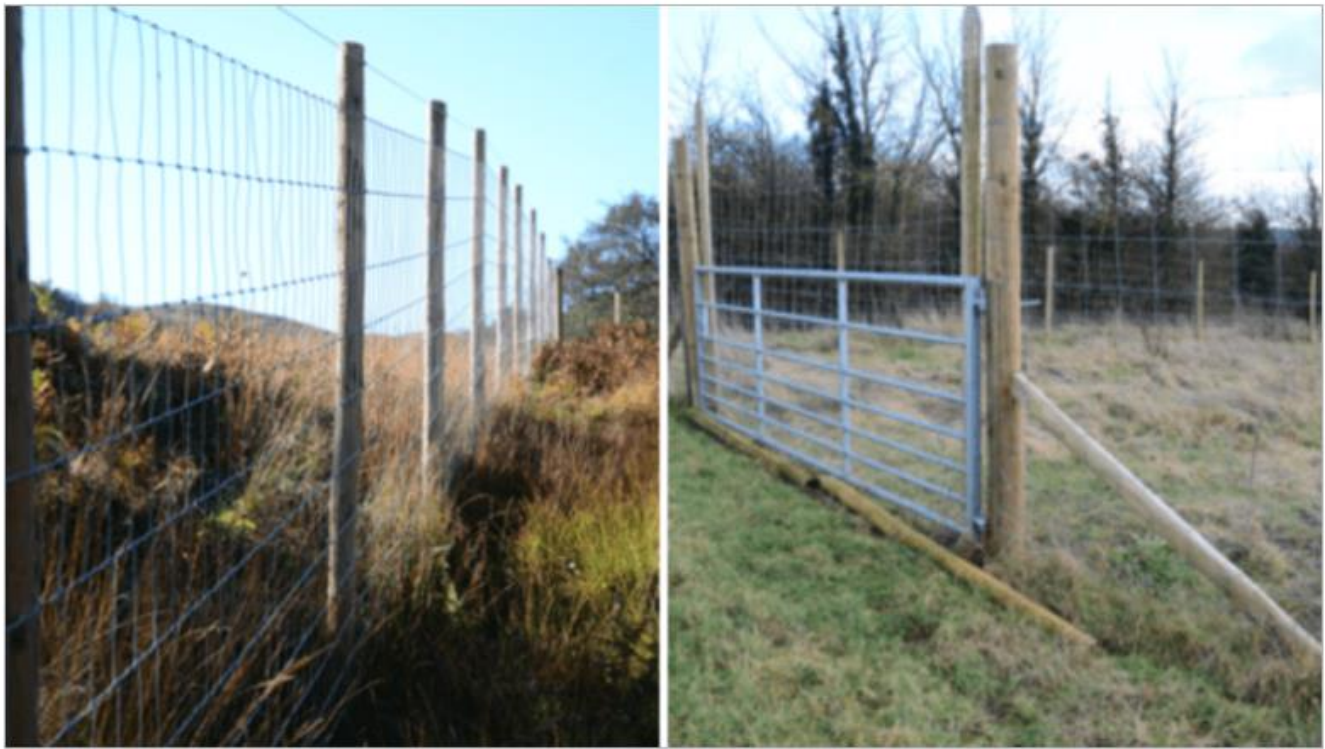
L to R: A well-maintained upland deer fence. Lowland deer fence and secure gate, plus rabbit mesh. Image credits: Mark Malins
